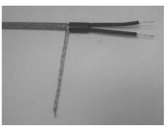
Crimp tube 9/3, L=20 mm is pulled in over the two conductors, all the way to the twisted screen in order to cover approx. 10 mm of the primary insulation and approx. 10 mm of the conductors.
