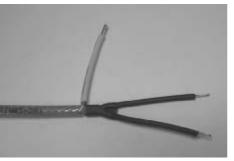
9. Now the heating cable is ready for direct connection.
