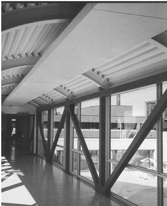
**FIGURE 4.11** Visible radiant hydronic ceiling panel system.
