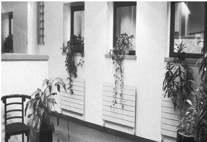
**FIGURE 2.20** Low-temperature electric or hydronic wall surface mounted radiant panels.
