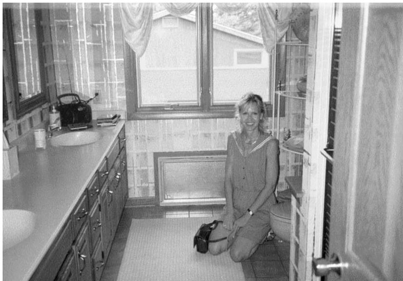
**FIGURE 2.18** Flat ceramic or glass panel recessed wall heater. (Photo courtesy of Radiant Electric Heat.)
