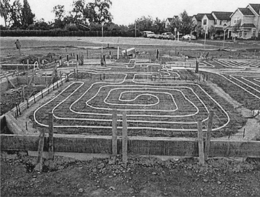
**FIGURE 1.4** Floor cooling.
