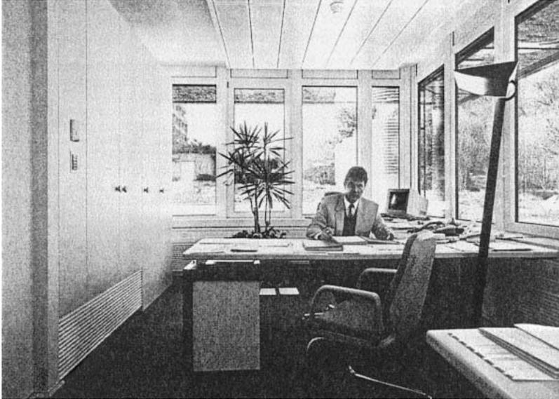
**FIGURE 2.6** Hydronic radiant ceiling cooling panels with displacement ventilation system.
