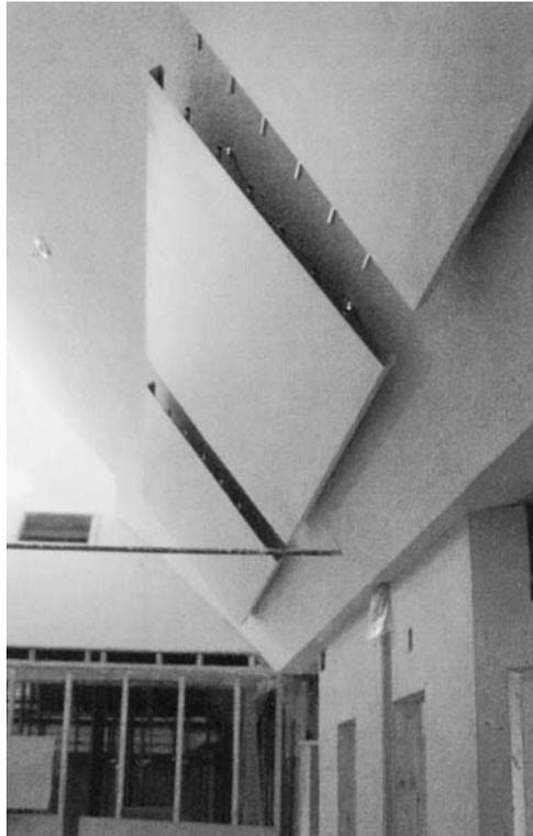
**FIGURE 1.15** Radiator panels, shown mounted on the cathedral ceiling, provide both heating and cooling.
