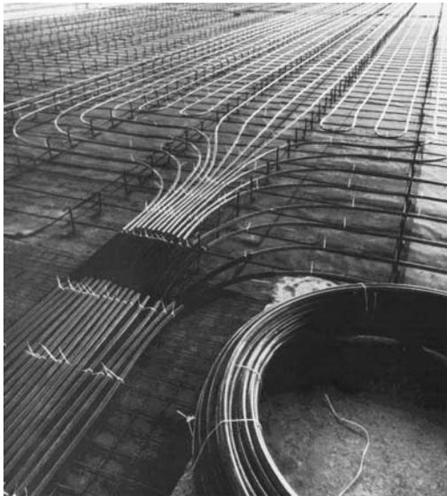
**FIGURE 4.14** Large, high-mass radiant hydronic floor installation. (Photo courtesy of Watts Heatway.)
