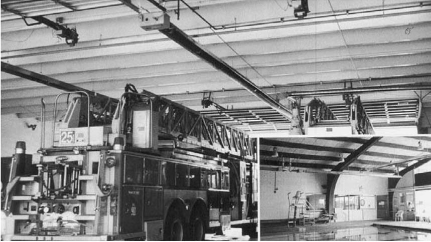
**FIGURE 2.3** Industrial gas-tube heaters. (Source: Photo courtesy of Detroit Radiant Products.)
