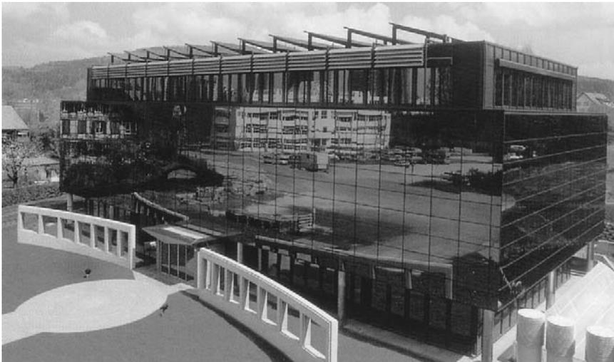
**FIGURE 1.3** Berne office building with cold façade, alternative energy generation, and chilled ceilings.
