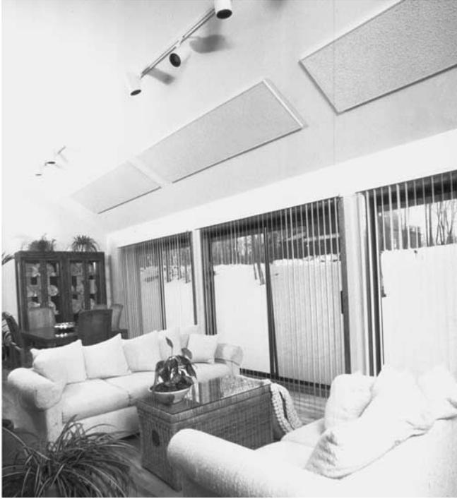
**FIGURE 2.7** Electric radiant ceiling panel. (Source: Photo courtesy of SSHC, Inc., Solid-State Heating Division.)
