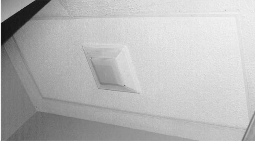
**FIGURE 3.1** ENERJOY Bathroom Comfort Center heat panel, with a centered exhaust fan, light, and night-light. (Photo courtesy of SSHC, Inc.)
