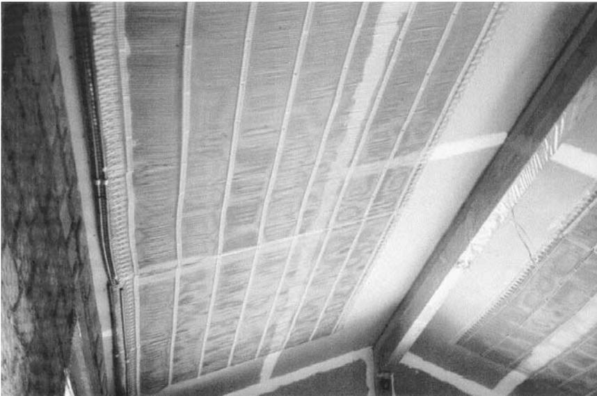
**FIGURE 4.10** Capillary radiant ceiling panel system.
