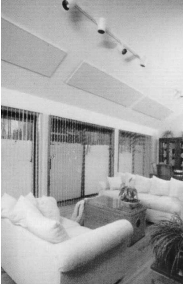
**FIGURE 2.7** Surface-mounted panels used for primary heating.
