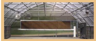
The Glacier-Cor PVC Cooling System is a complete evaporative cooling system with a 3' high wall and 4" pads. It works together with your greenhouse fans to lower temperatures 10-25 degrees. The sump is built-in and eliminates the need for a separate external sump tank, minimizing the amount of piping needed for the system.
