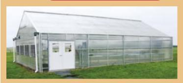
Our 30' x 60' **California package** is designed for horticulture programs that want the same features as the Texan with a smaller structure. Besides the size the only difference is a 3' x 25' wet wall, 3 motorized inlet shutters and 4 horizontal air flow fans. *Everything else is the same*.
