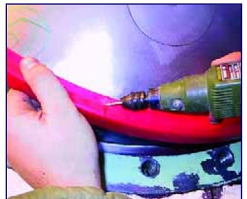
Installation of giant seal kit (welded and adapted)
