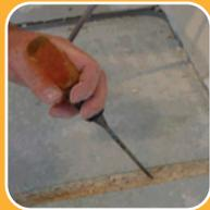
1. After preparing a smooth surface, create a groove in the floor to accommodate the conduit for the floor probe.
