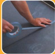
2. Measure the area to be heated and fit the Ecomax-Lite Thermal insulation to the floor securely following the manufacturers instructions.
