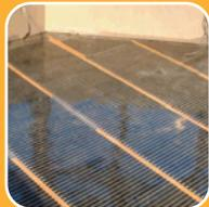
3. Roll out the lengths of EcofilmSet and trim to length along cutting line as required. Insulate trimmed ends as per instructions before taping the elements into position, taking care to locate the "cold tails" on the wall nearest the thermostat connection box.
