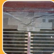
5. Tape over the cap ends and cables so that they do not move out of position.
