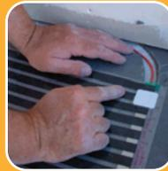
4. Cut away sections of the insulation to accommodate the white sealing caps and cables of the element strips as well as the area where the floor probe will be located.
