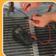
6. Check individual element length resistance using an Ohmmeter. Insert the thermostat floor probe into the protective conduit. A fully qualified electrician must now make the final connections to the mains supply & install the thermostat.
