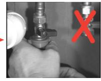
If the appliance is cold fill only, connect the hose to the cold tap and leave the hot tap (if there is one) unconnected and switched off.
