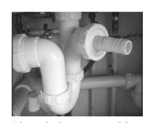
Alternatively you may wish to connect the Drain Hose to a sink spigot. Ensure the spigot is clear if this is the first time it has been used.
