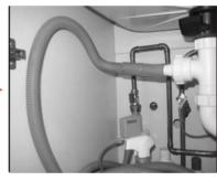
Both the above type Drain Hoses will fit onto a spigot as they are tapered to grip the hose. Position the hose with a loop at the top to ensure correct drainage.
