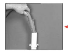
If your Drain Hose looks like this you do not require the «U» piece. Just push the hose firmly into the standpipe.
