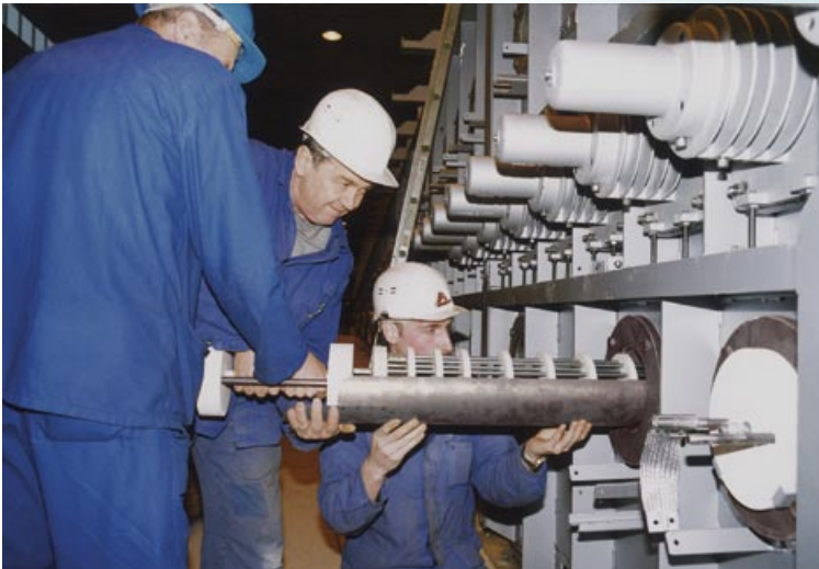
Installation of Tubothal and PM tubes in a continuous annealing line
