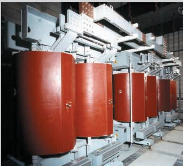
Transformer for electrical stirring (10 MVA).
