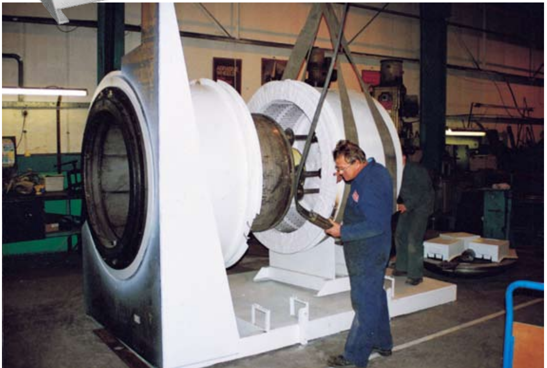
Fig. 30 Assembly of FIBROTHAL ROB-segments for a vacuum purge furnace
