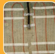
6. Insert the floor probe into the tubing and ensure the probe is between two cables. Test the cable resistance reading. A fully qualified electrician must now make the final connection to the mains supply and install the thermostat.
