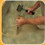
1. After preparing a smooth surface, measure the area to be heated. Fit the Ecomax Insulated Tile Backer Board to the floor securely following the manufacturers instructions. Create a groove in the board to accommodate the conduit for the floor probe.
