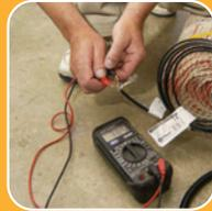
2. Check the cable resistance using an Ohmmeter before beginning the layout.
