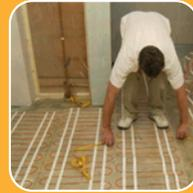
4. Once you are satisfied with the proposed layout stick the matting to the floor using the integral self-adhesive fixing strips.
