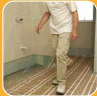
3. Planning is extremely important at this stage so it is advisable to lay the mat out over the surface of the floor without sticking it down to enable you to have a clear idea of how the mat will be laid.
