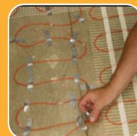
5. For hard to reach areas or areas where the mat cannot be fully rolled out, detach the cable from the mat and attach to the floor uniformly with duct tape.
