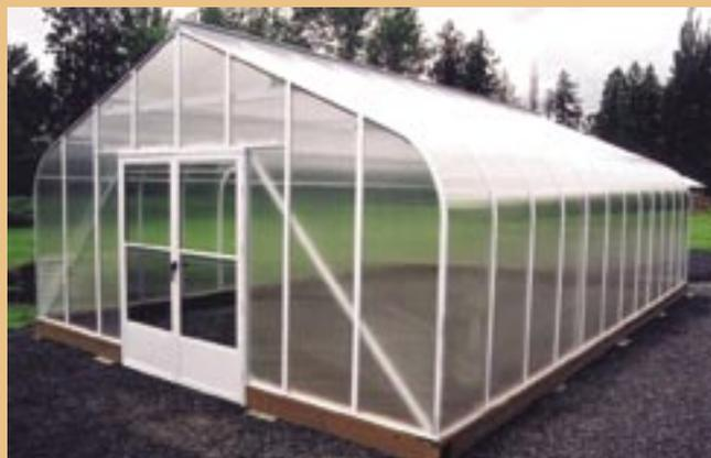
This aluminum frame is also available with a curved-eave and can be covered with glass or polycarbonate or both.
