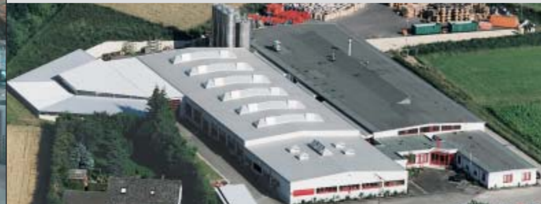
Research & production centre in Windsbach
