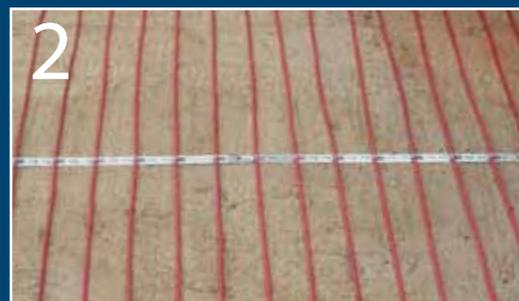
The fixing strip is laid at regular intervals across the floor using either masonry nails or tape, which ensure s that the cable can be evenly spaced. The cable can either be laid on a concrete base or foil backed insulation.
