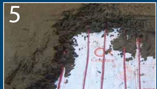
The heating cables are covered with sand and cement screed. Once the screed is dry, the heating should be turned on gradually over a 48 hour period.
