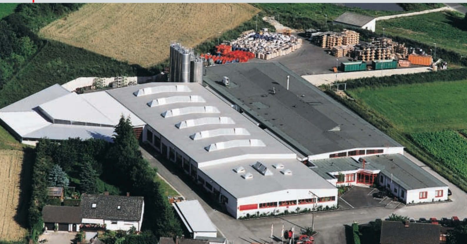
Production Windsbach / Germany
