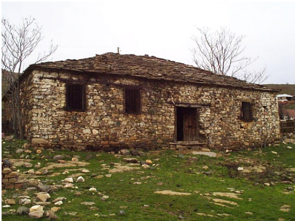
Photo 3.2 Home in Dolno Orehovo. The home is typical of the style found on the Pelagonia plain but is constructed of stone due to the village being situated on the fringes of the Mariovo hills
